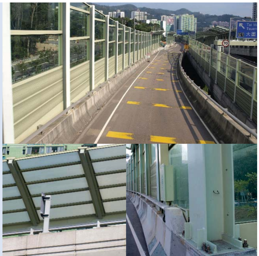
Shatin New Town Stage II, Road T3 and Associated Works (ST79/02) T3號道路及相關道路工程
