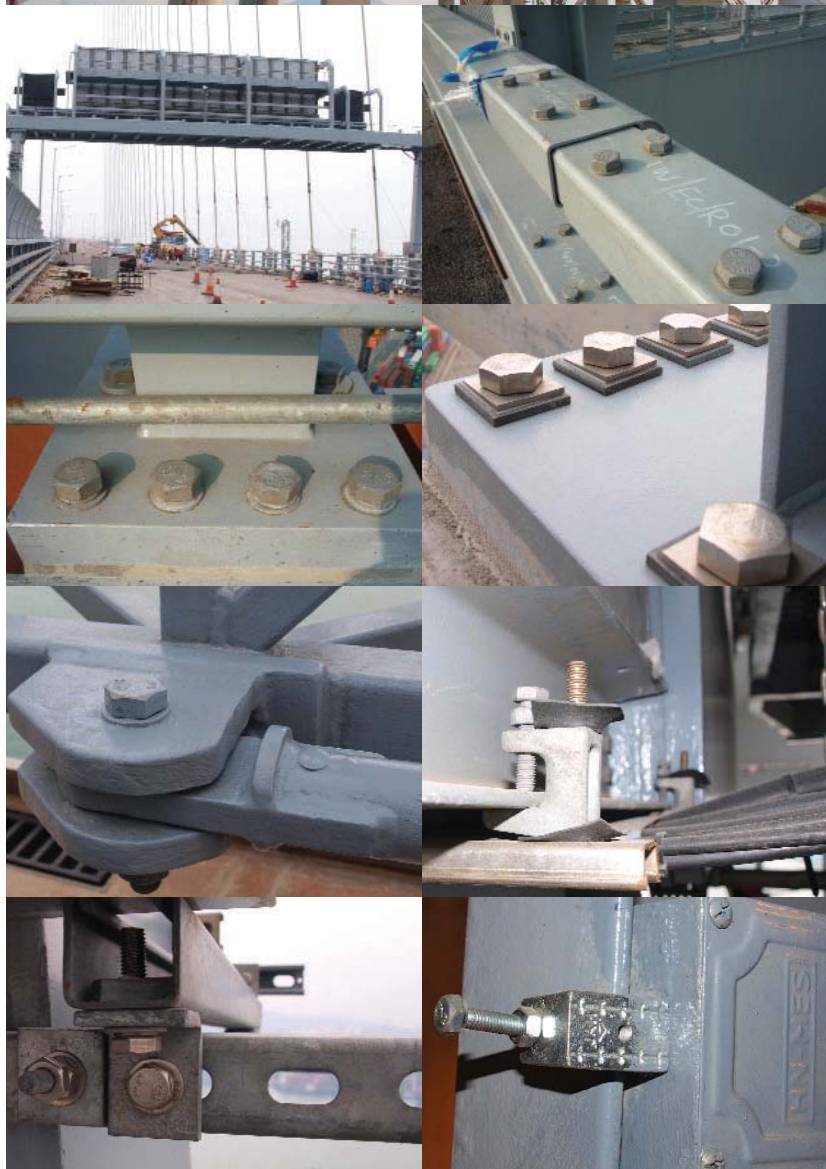
Route 8 - Stonecutters Bridge (HY/2002/26)
